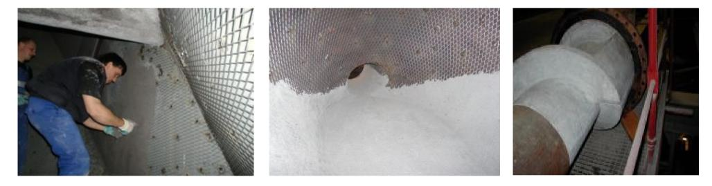
Very good for protection against minerals in sliding contact with steel, eg. Chutes, Pipelines, Vertical mill outlets, Filter inlets.
