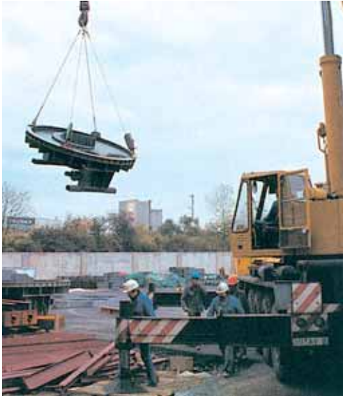
Lifting of workshop mounted main CENTREX™ components on site
