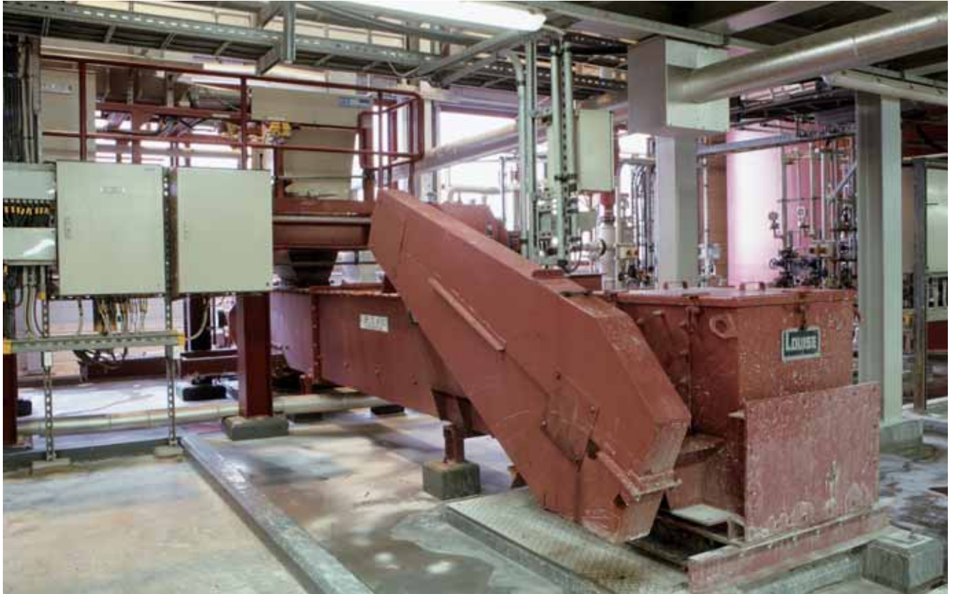
LOUISE Double-Strand Chain Conveyor, feeding 2 silos
